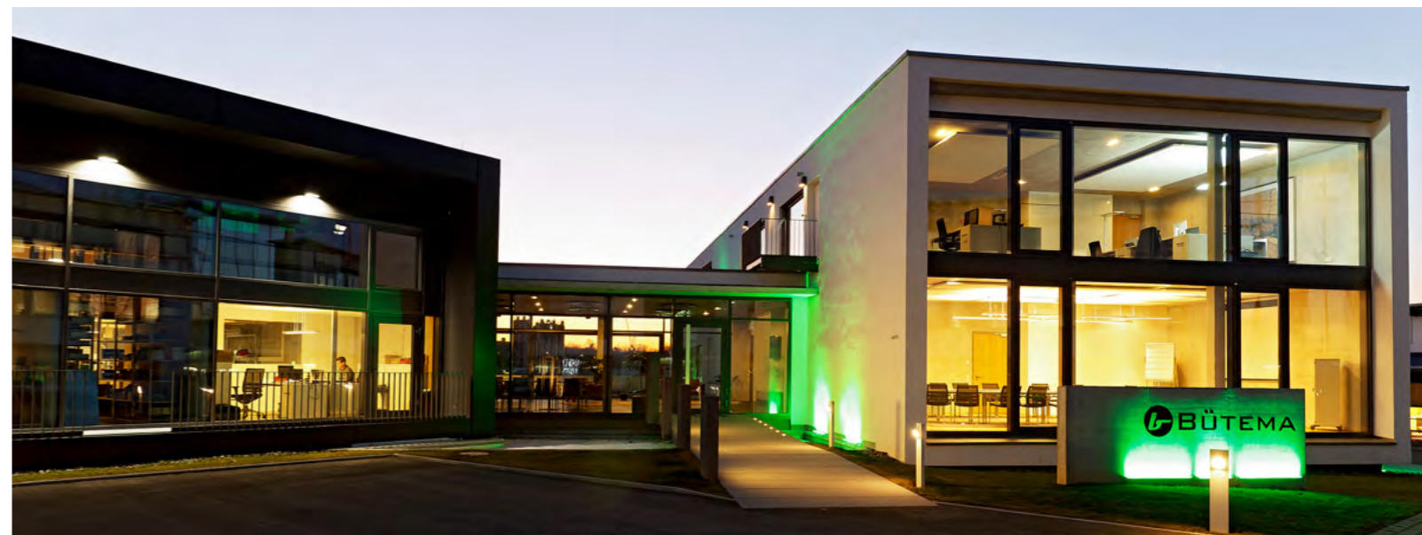
Bütema AG Headquarter in Bietigheim-Bissingen
